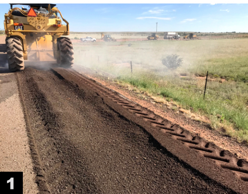
Falling Asphalt Mixed into Base
