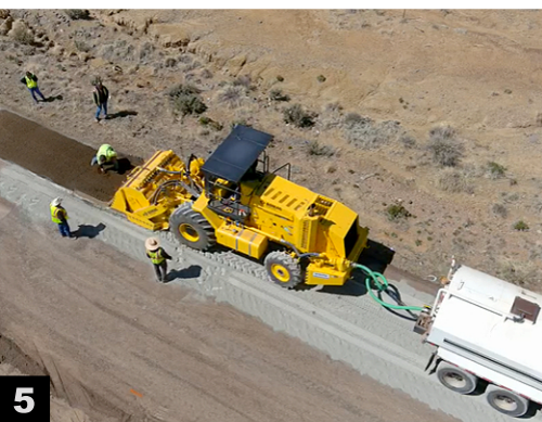
Mixing LithTec™ into the Base
