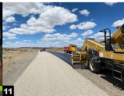
Applying Chip Seal (or Asphalt)
