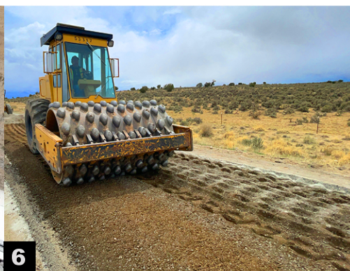
Sheepsfoot Compaction at OMC
