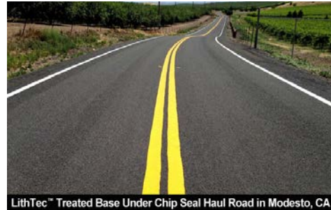
LithTec™ Treated Base Under Chip Seal Haul Road in Modesto, CA
